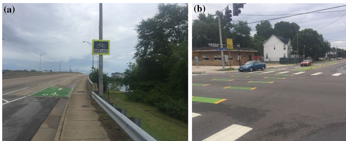
Fig. 10 Cycling lanes introduced into Norfolk, VA that overcome the geographic limitations of a bridges, and b complex historic road layouts
